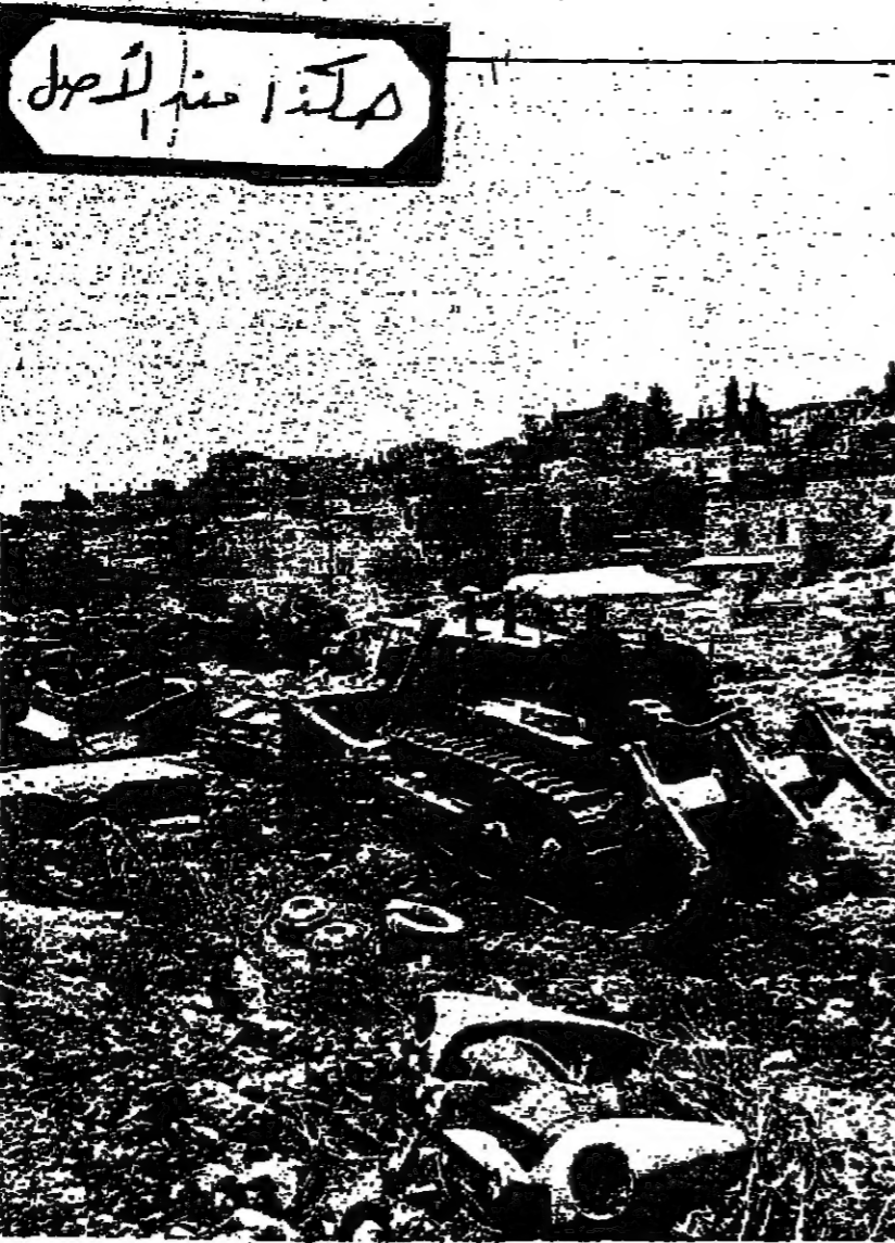
END OF AN EYESORE: Bulldozers have begun clearing the scrap heaps in Wadi Joz, Jerusalem. (Sunday)
